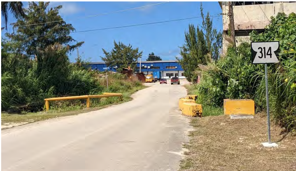
Photo 6-17 Existing Condition: Narrow Culvert on Route 314, West of Route 30 (Saipan)
