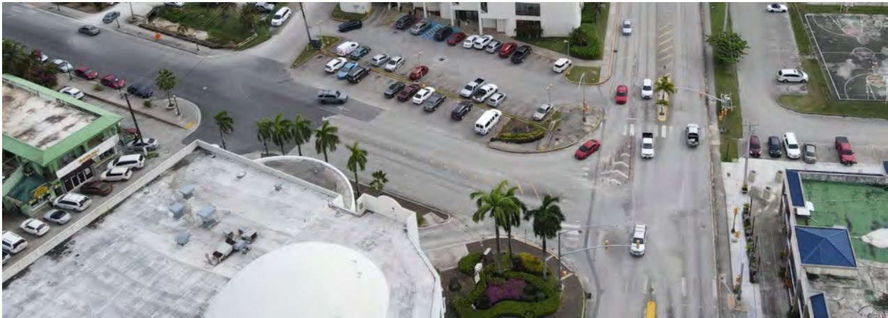
Photo 6-23 Existing Intersection (Southbound View)
