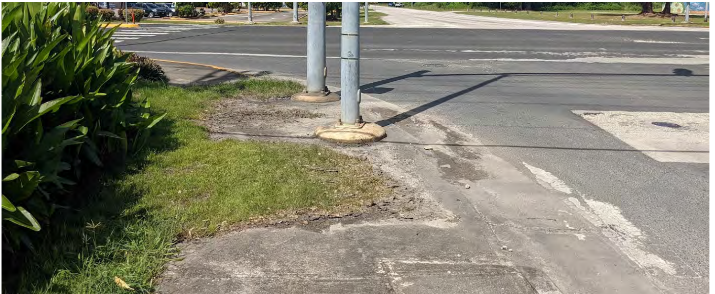
Photo 6-38 Existing Condition: Missing ADA Curb Ramps at Intersections (at Middle Road/Chalan Pale Arnold)
