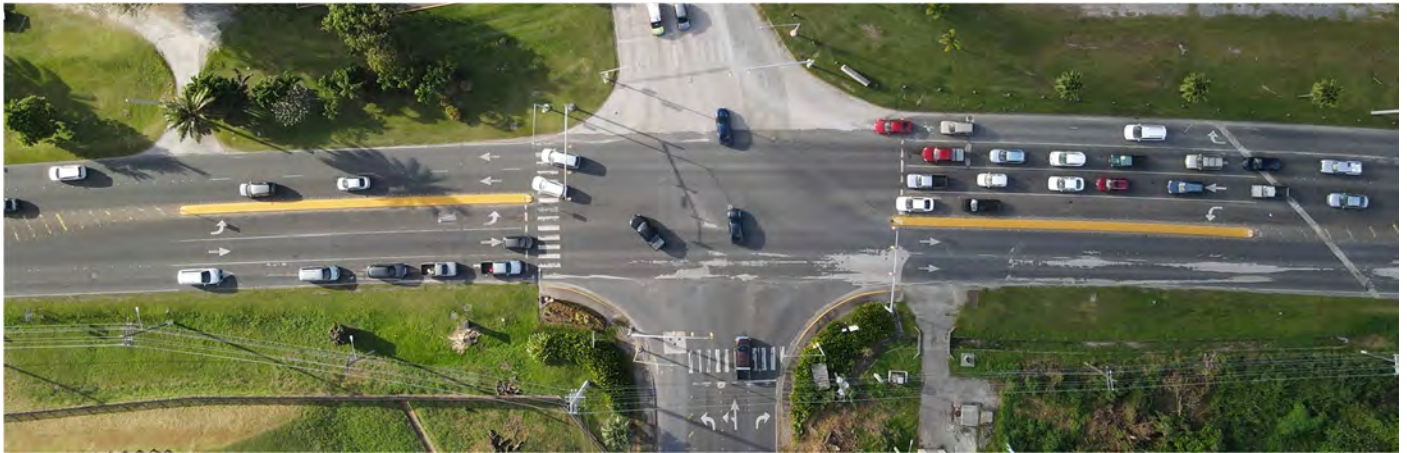
Photo 6-14 Example of an Existing Traffic Signal: Route 30 & Route 38 (Saipan)
