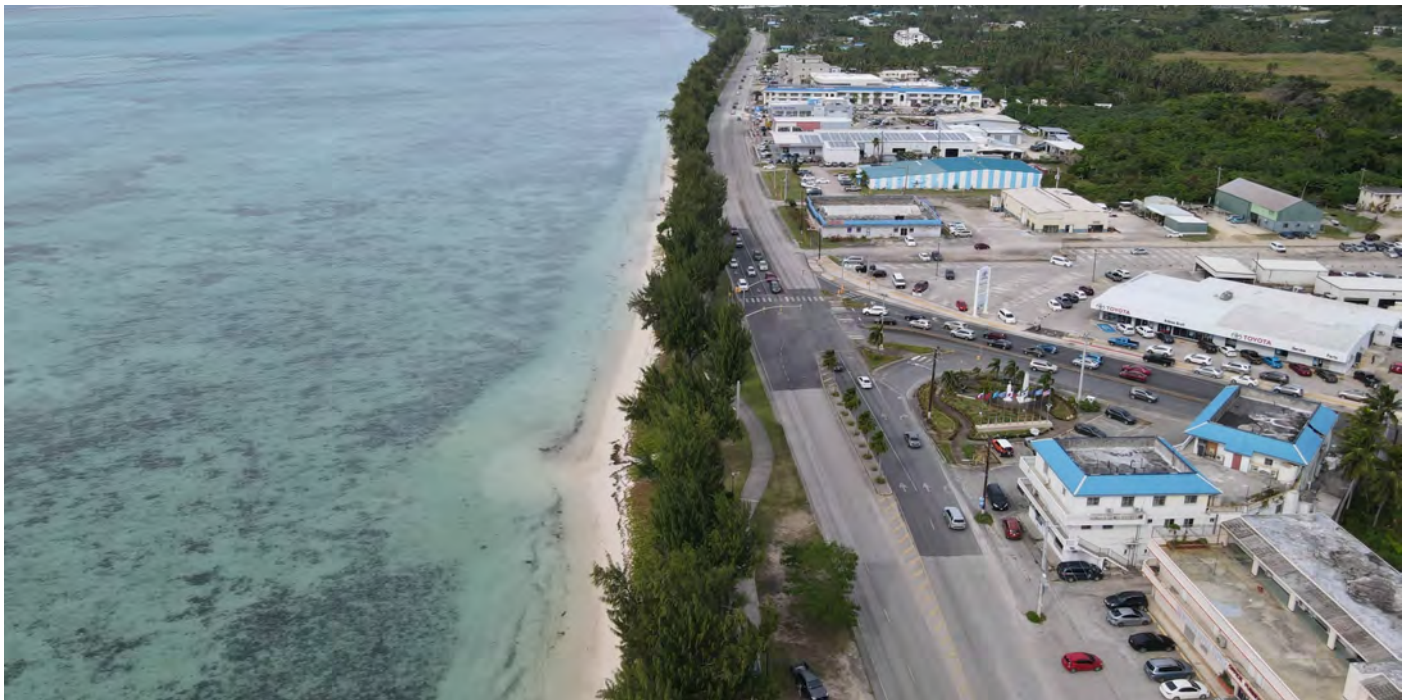
Photo 6-53 Beach Roadway Parkway
