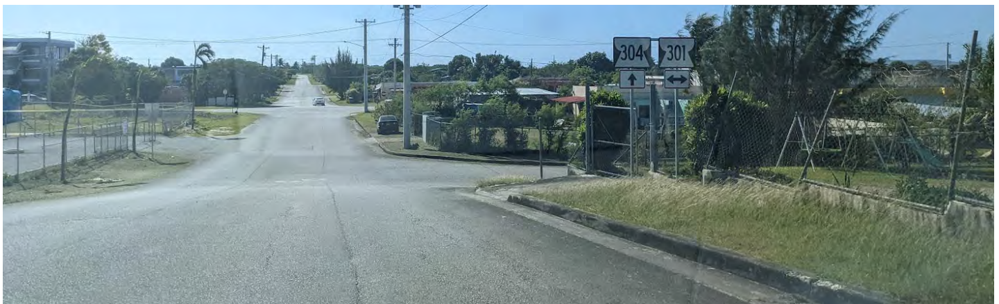
Photo 3-8 Lack of Pedestrian Facilities near a School (Intersection of Route 304 & Route 301)
