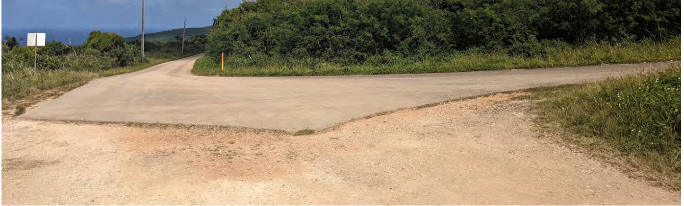
Photo 6-13 Existing Condition: Blind Curve on Route 318 (Saipan)
