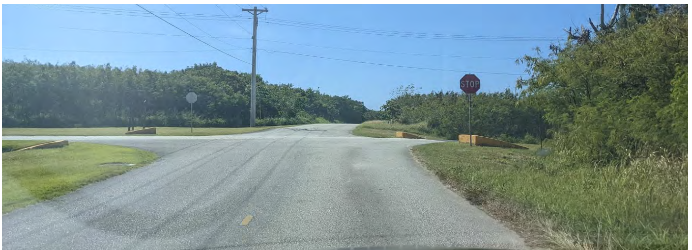
Photo 6-26 Existing Condition: Southbound Approach
