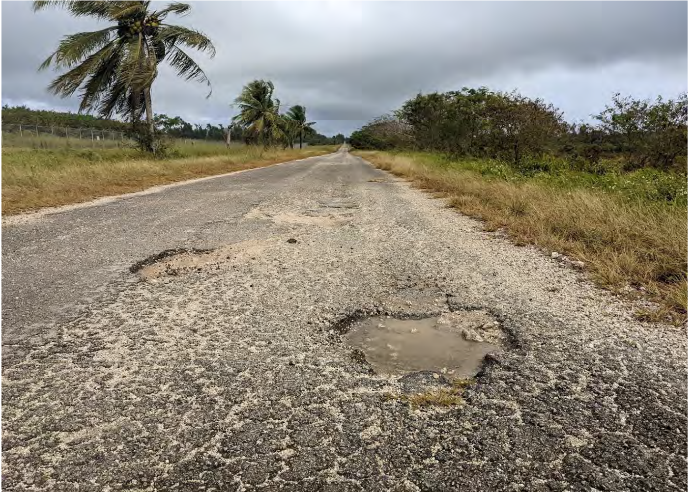
Photo 6-56 Existing Pavement Condition on Route 21 (Broadway)
