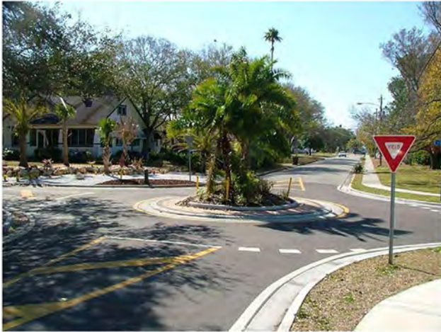
Figure 3.8.1. Small Modern Roundabout (Source: Ken Sides)
