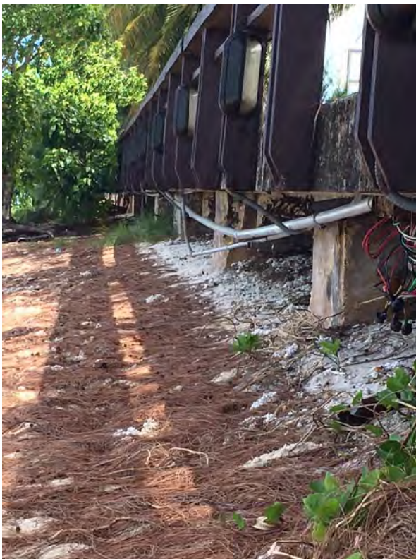
Photo 3-1 Existing View of Beach Road Parkway (A)
