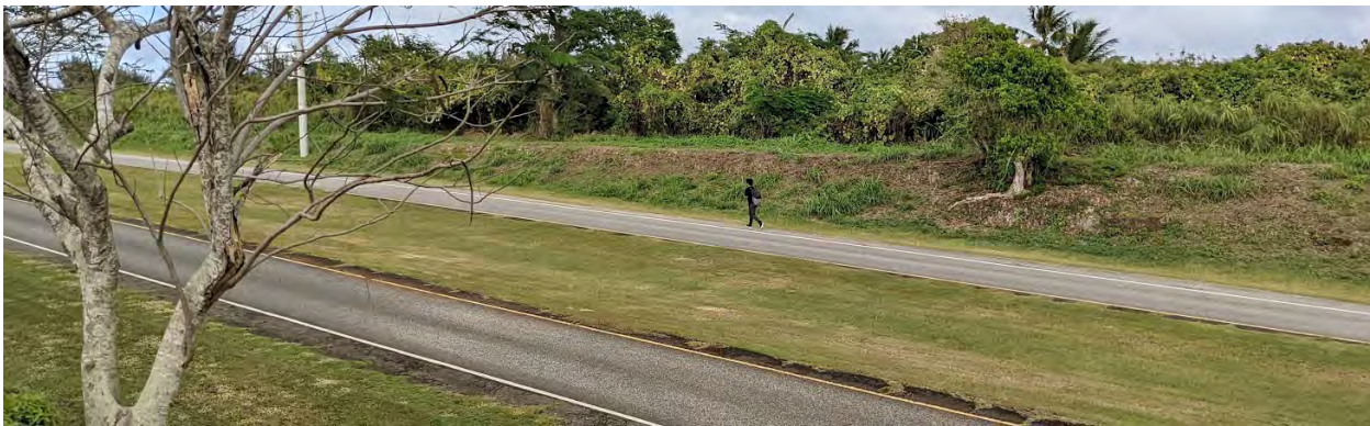
Photo 6-8 Lack of Pedestrian Facilities on Route 21 (Broadway) (Tinian)
