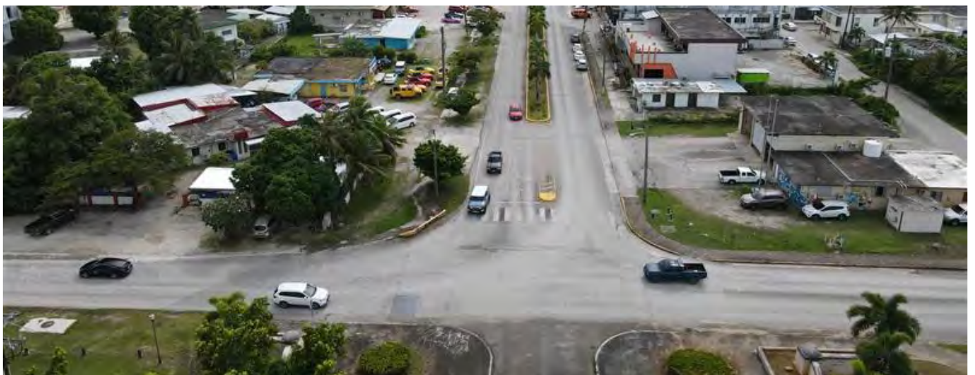
Photo 6-31 Existing Intersection – Southbound View
